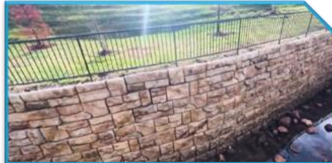
Gravity Wall with Safety Railing
