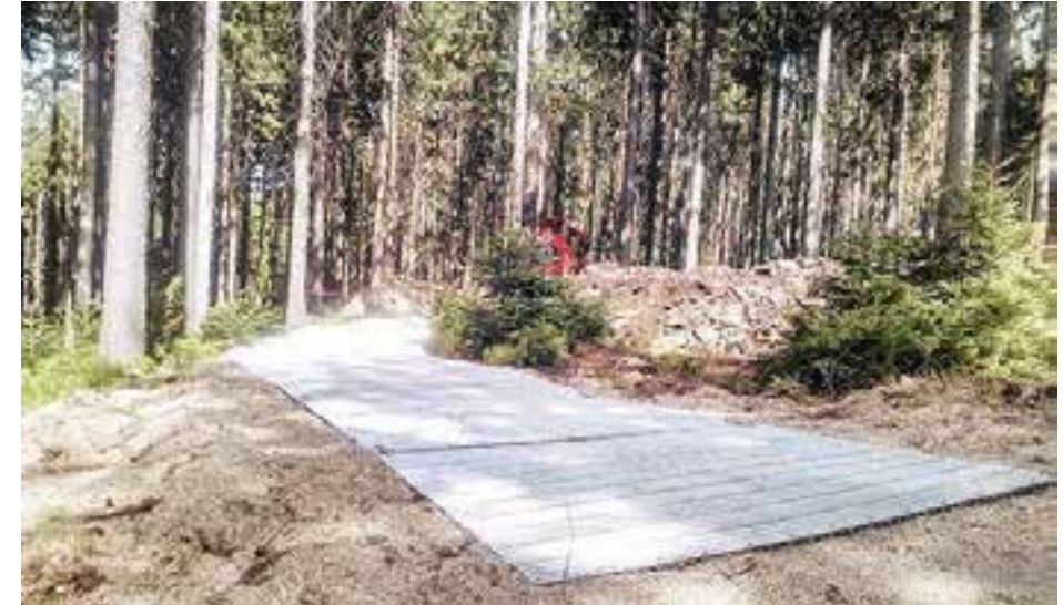
Deck Mat/Construction Access Road
